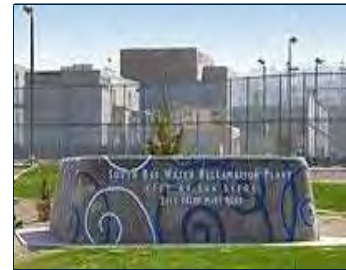
South Bay Water Reclamation Plant
