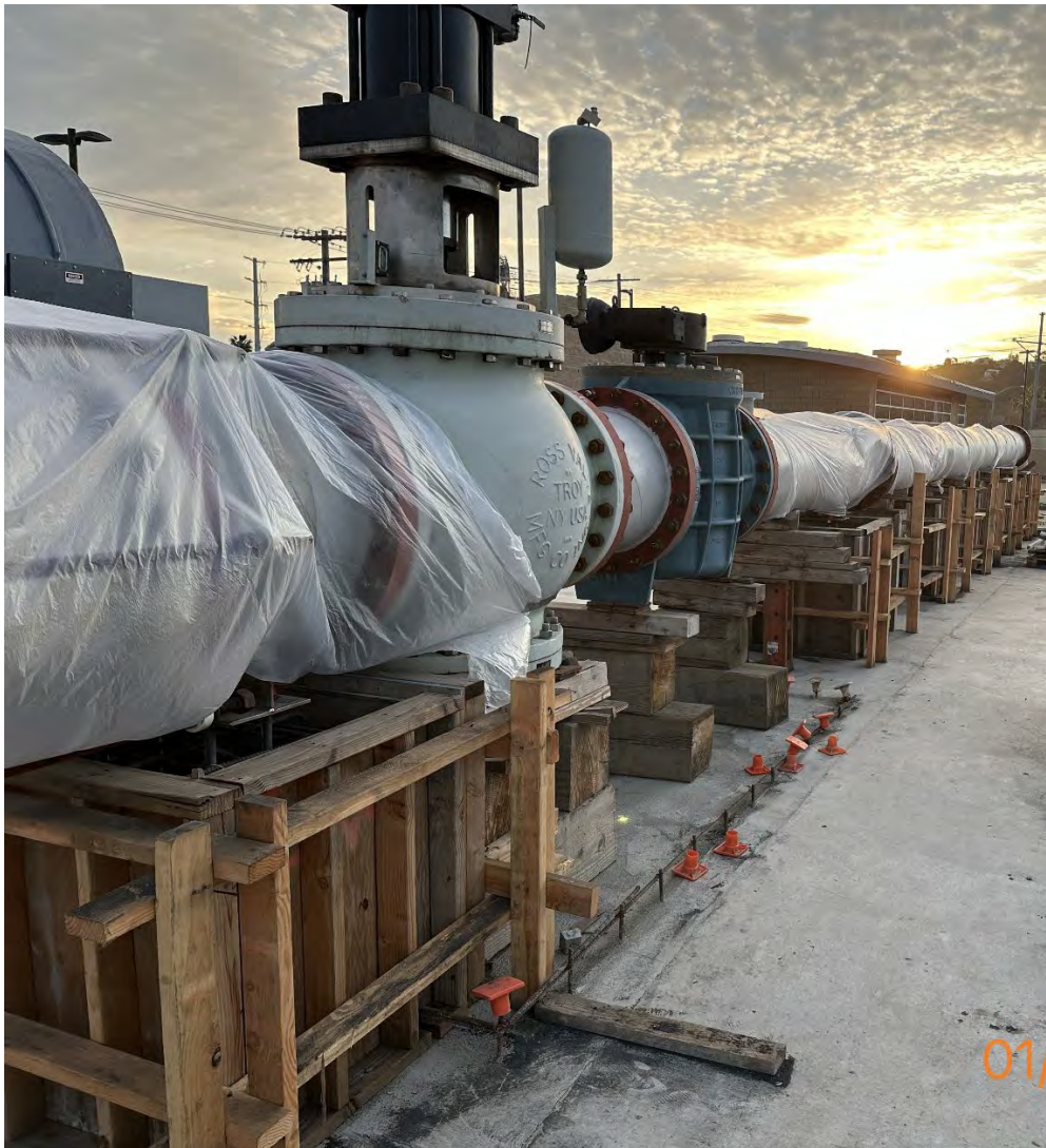
Morena Pump Station Roof – Pipe Supports – January 2026
