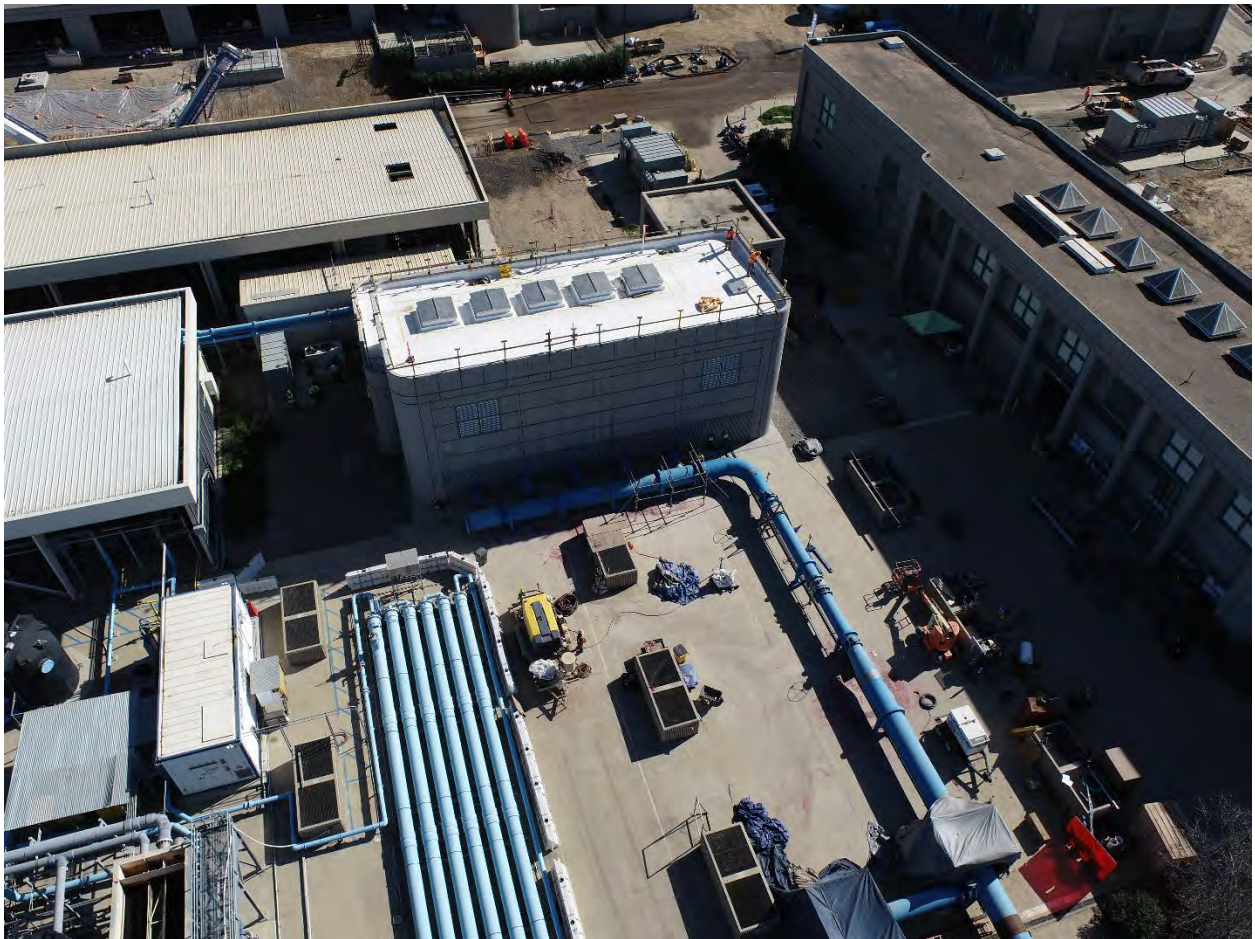
North City Water Reclamation Plant Expansion – January 2026 NCPWF Influent Pump Station
