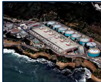
Point Loma Wastewater Treatment Plant
