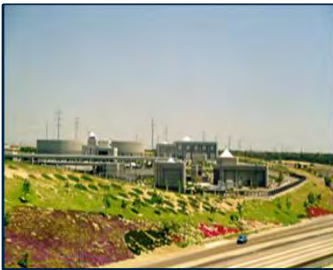
North City Water Reclamation Plant
