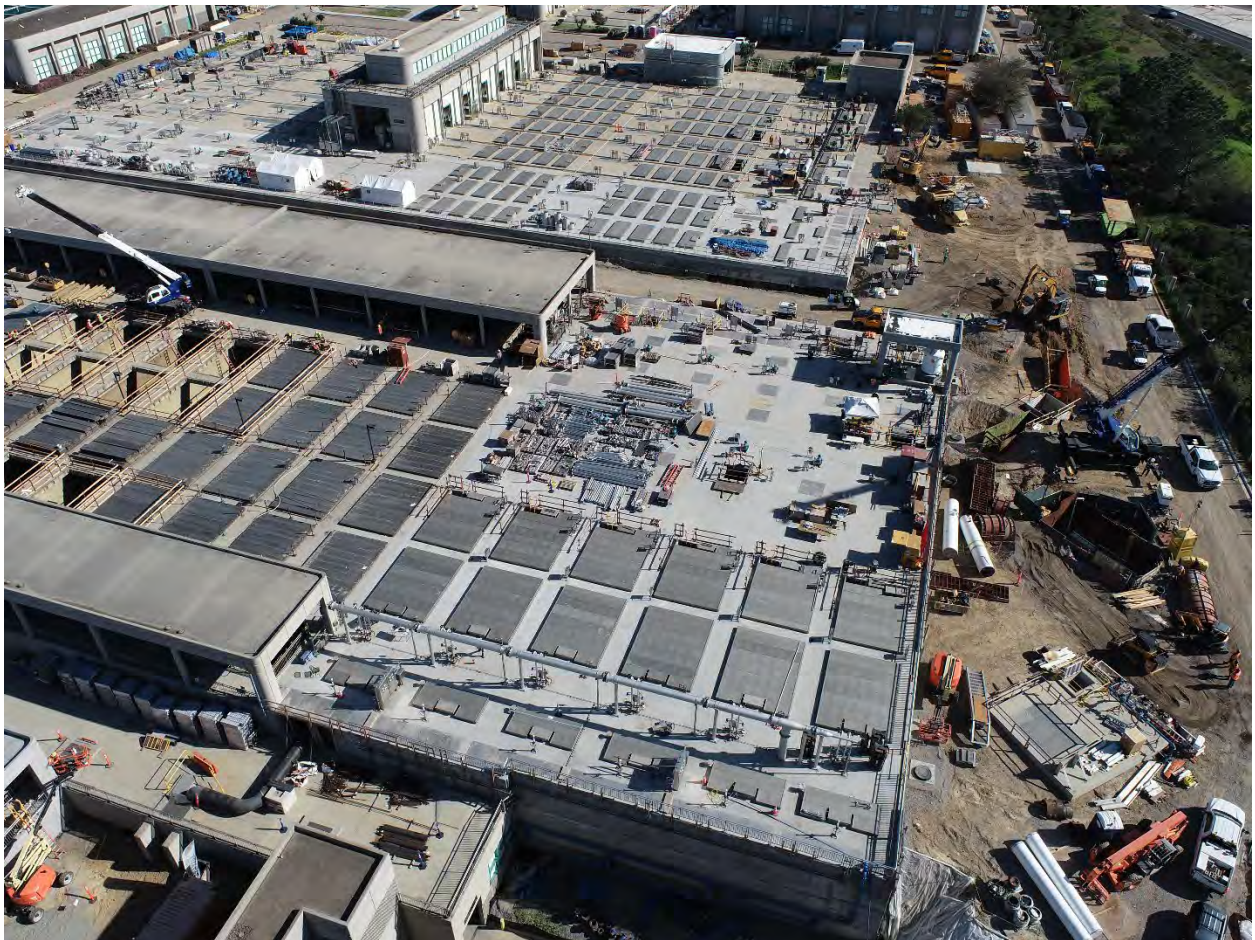
North City Water Reclamation Plant Expansion – January 2026 Second Stage Bioreactor Basins
