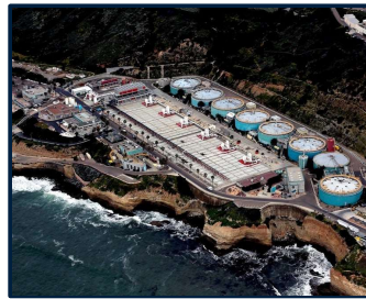
Point Loma Wastewater Treatment Plant
