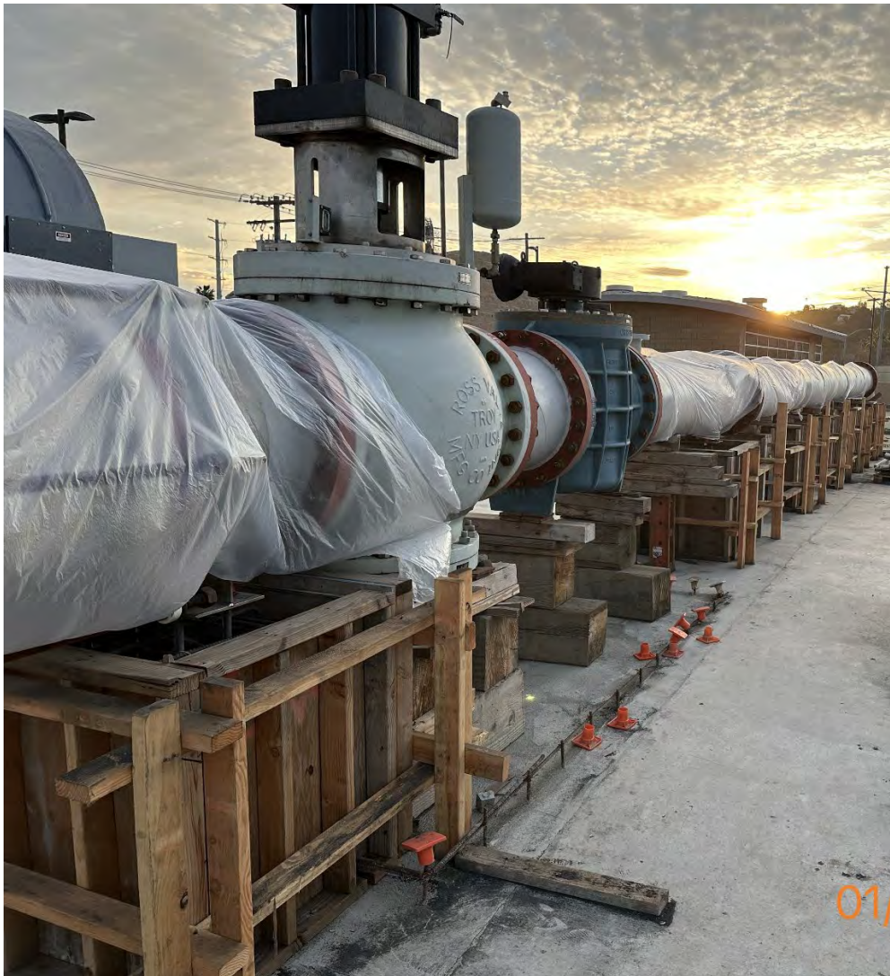
Morena Pump Station Roof – Pipe Supports – January 2026
