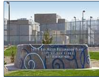
South Bay Water Reclamation Plant
