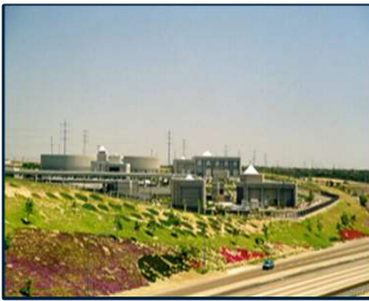
North City Water Reclamation Plant
