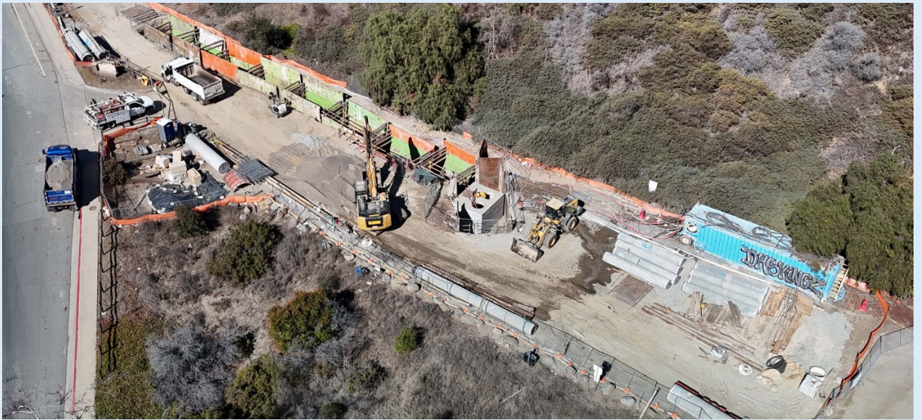
San Clemente Launch Shaft to Open Cut Casing. February 2025
