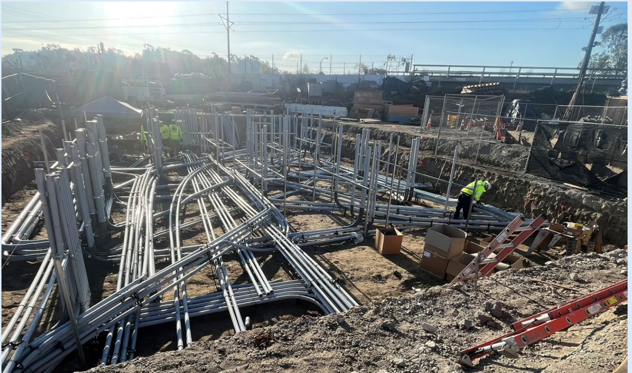
Morena Pump Station Electrical Building Conduit Placement
