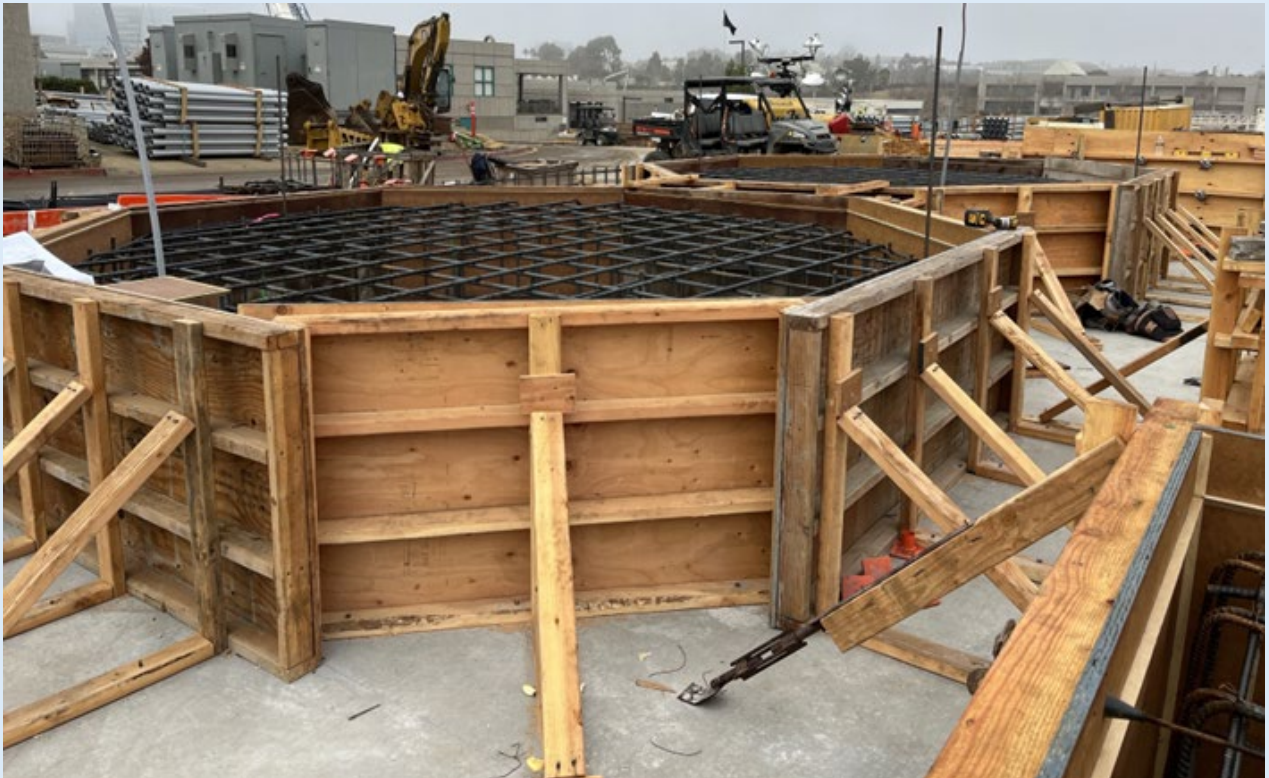
North City Water Reclamation Plant Expansion – February 2025. Carbon Chemical Facility: Forming Chemical Tank Pads
