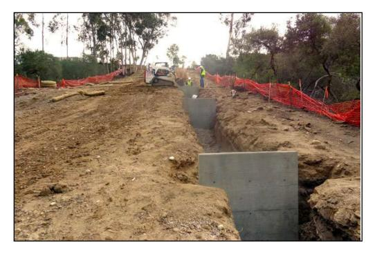
The Scripps Ranch Reservoir, a source of water for the community, must be isolated, drained, and inspected every two years. The City conducted a study in March 2010 called the Scripps Ranch Reservoir Roof Bracket and Drain Slope Repair Planning Study. The study found that water conveyed out of the 18-inch storm drain on the north side of Spring Canyon Road had eroded the canyon slope. The storm drain, therefore, needed to be replaced and slope repaired.
