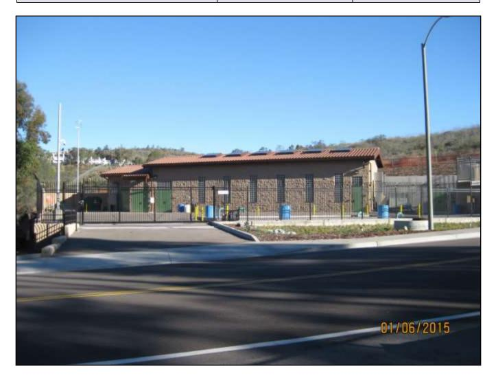
The Scripps Miramar Ranch Pump Station supplies over 90% of the water to the Scripps Ranch Service Area and all of the water to portions of Scripps Ranch. This project replaced the aging station. The project included design and construction of a facility to house six large turbine pumps and electrical controls for the station, installation of equipment, connection to three existing pipelines, equipment testing, parking and space for a trailer-mounted emergency generator.
