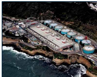
Point Loma Wastewater Treatment Plant
