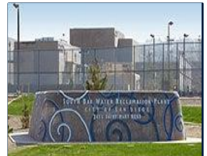
South Bay Water Reclamation Plant
