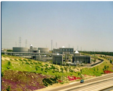
North City Water Reclamation Plant
