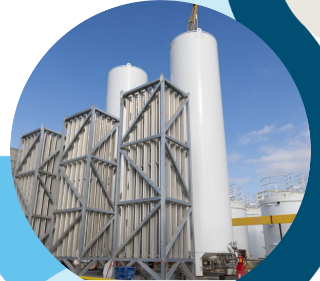
oxygen tanks at the Pure Water facility under construction
