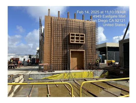
North City Water Reclamation Plant Expansion – February 2025 Update NCPWF Influent Pump Station: Installing Wall Rebar.
