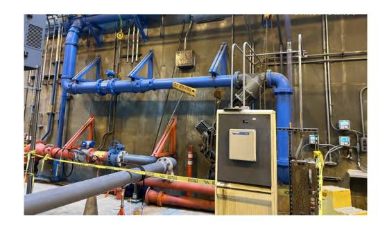
North City Water Reclamation Plant Expansion – February 2025 Update Effluent Pump Station: Work ongoing for 8"/10" UWHP.
