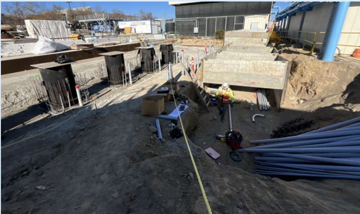
North City Water Reclamation Plant Expansion – January 2025. NCPWF Influent Pump Station: Under slab conduit installed and CLSM poured. Bulkhead construction moving forward.
