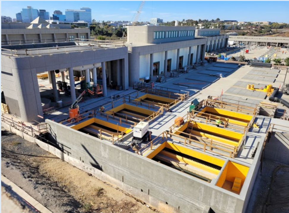
North City Water Reclamation Plant Expansion – December 2024. Primary Sedimentation Basins: Basin 7 and 9 Quantitative hydrotesting began this week.
