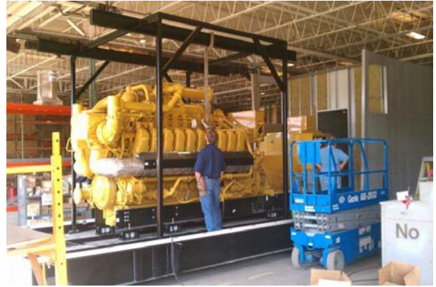
New cogeneration engine, capable of producing 1600 kW of power
