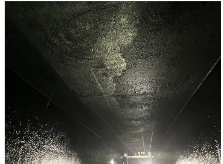
PHOTO 2: VIEW DOWN WET WELL 1 FROM ABOUT 30' EAST OF INTAKE TO PUMP 4
