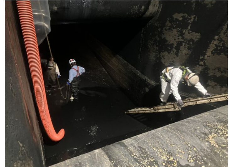
PHOTO 1: DESCENT FROM SLUICE GATE LEVEL (EL -28) TO SUMP LEVEL (EL -41)
