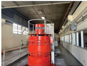
Pump Motor – 6 Motors, Pump Control Room to Right, Removable Panels on Left to Extract Pumps and Valves
