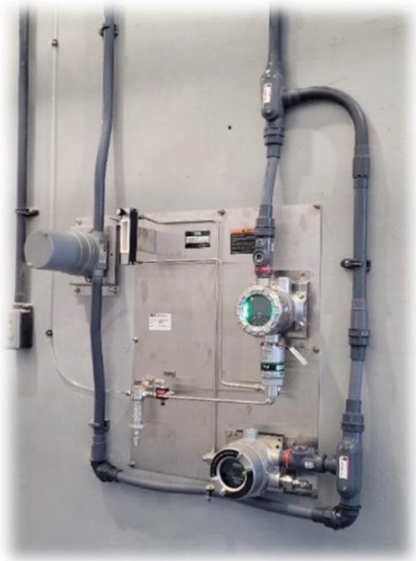
Figure 1. New wall mounted gas sensor in the pipe gallery.
