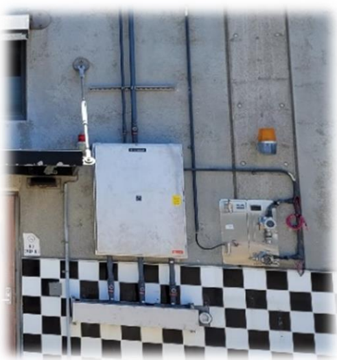
Figure 2. New outdoor wall mounted gas sensor.
