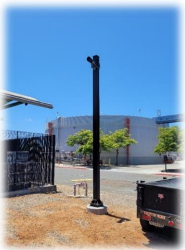
Figure 3. New pole mounted gas sensor.
