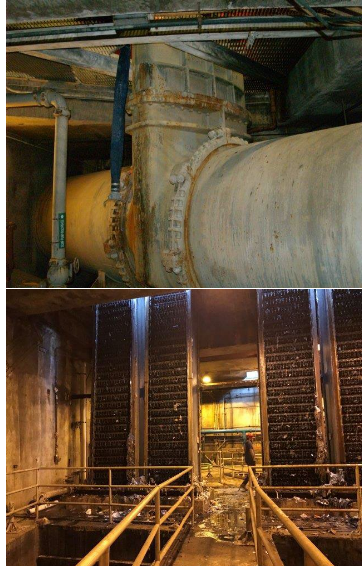
Pump Station 2 - suction valve (upper) screens below grade (lower).
