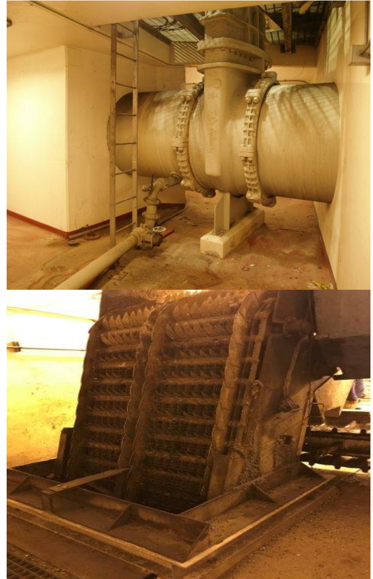
Pump Station 1 – suction valve (upper) and screens (lower).
