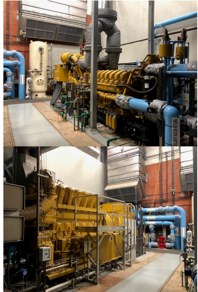
New Natural Gas Engine Generator (upper)
