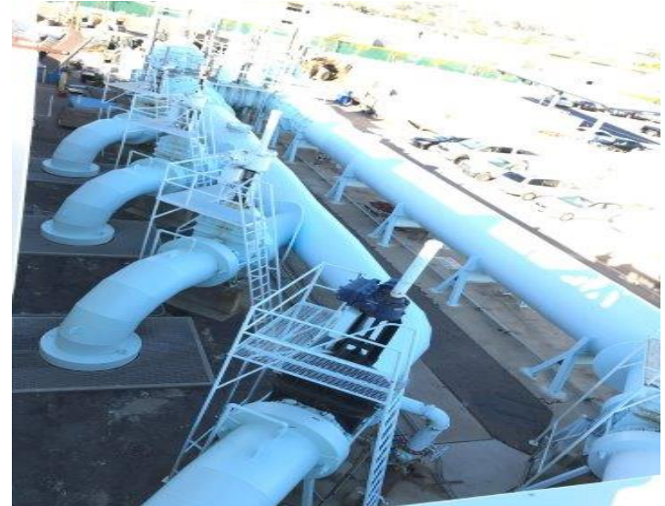
Pump Station 2 – suction valve (upper) and discharge header (lower).
