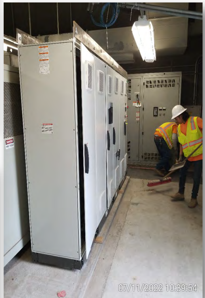
Photo 2. Crews installing new VDF.
