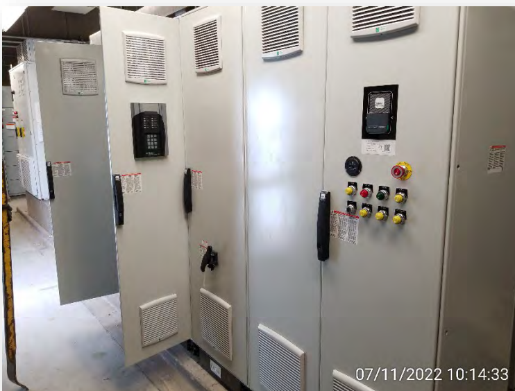
Photo 3. The new installed VDF.
