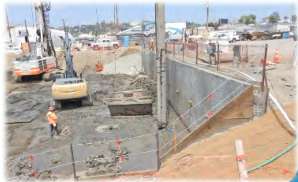
Stone Column Installation- May 23, 2022
