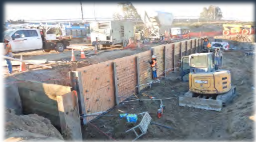
Beam and Lagging Shoring System Installation- March 1, 2022
