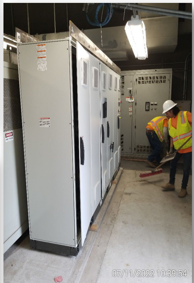
Photo 2. Crews installing new VDF.
