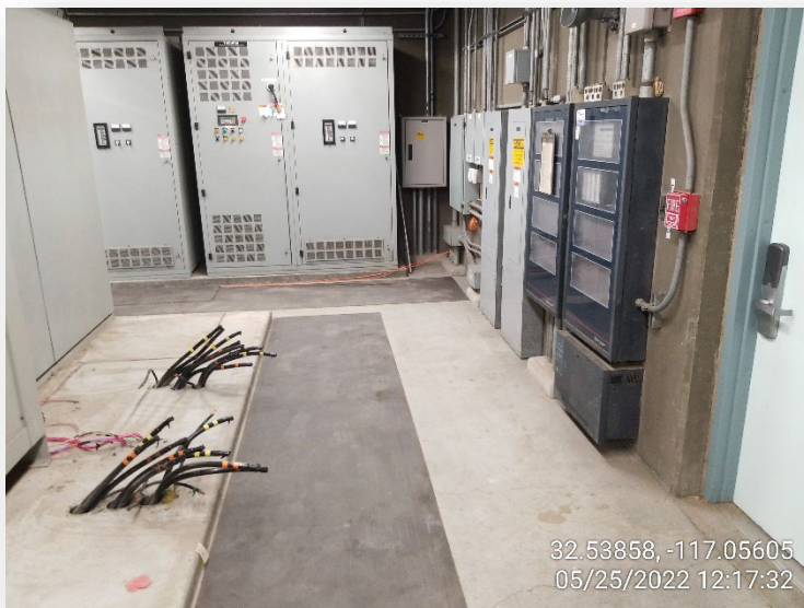
Photo 1. Removal of the old VDF.
