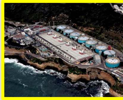
Point Loma Wastewater Treatment Plant
