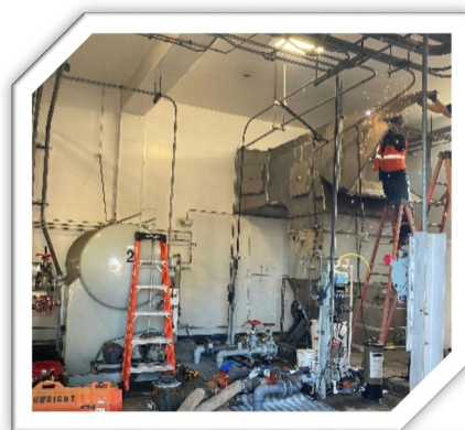
Photo 2. PS1 Existing duct demo using plasma cutters.
