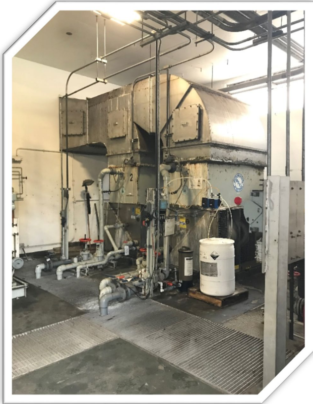
Photo 1. PS1 Existing cooling towers.
