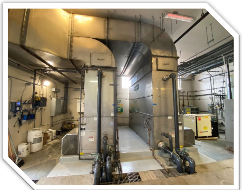
Photo 5. PS2 New cooling towers and chemical system.
