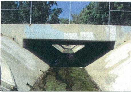
**Project 8: Pilot Concrete Channel Infiltration Project.** The *Pilot Concrete Channel Infiltration Project* will convert a portion of the concrete channel in Woodglen Vista Creek (and other channels as budget/logistics permit) to a more porous base, facilitating infiltration of dry weather flows without compromising flood control capacity. This effort will assist the City of Santee and other MS4 Copermittees in the attainment of bacteria TMDL waste loading allocations.
