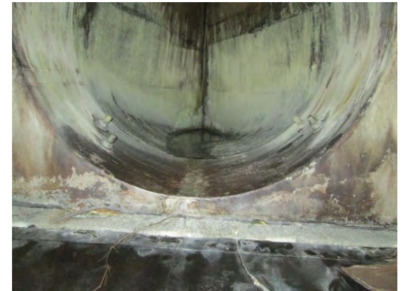
View of interior of 'duckbill' valve and overflow box structure.
