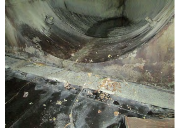
View of liner of overflow box structure.
