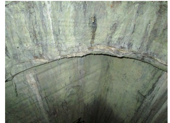
View of cuts in liner at bottom of short barrel section in manhole.
