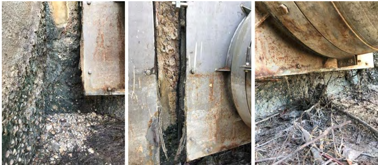
Figure 6. Duckbill Installation Plate Concrete Loss and Corrosion
