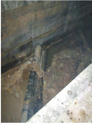
View of angled weir walls in main open channel.
