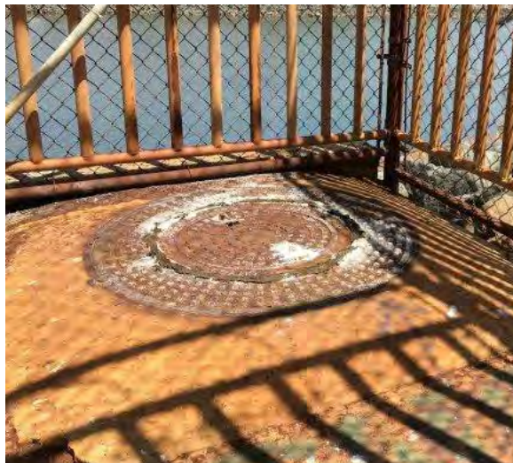
Figure 7. Corrosion of the South Transition Structure Manhole Cover
