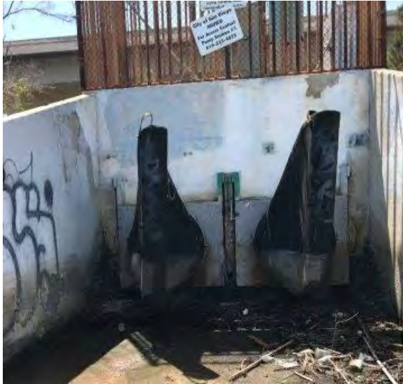
Figure 4. Spillway Duckbill Valves
