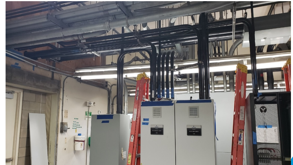
Installation of Control and Signal Conduit Rough-Ins – 06/18/2020
