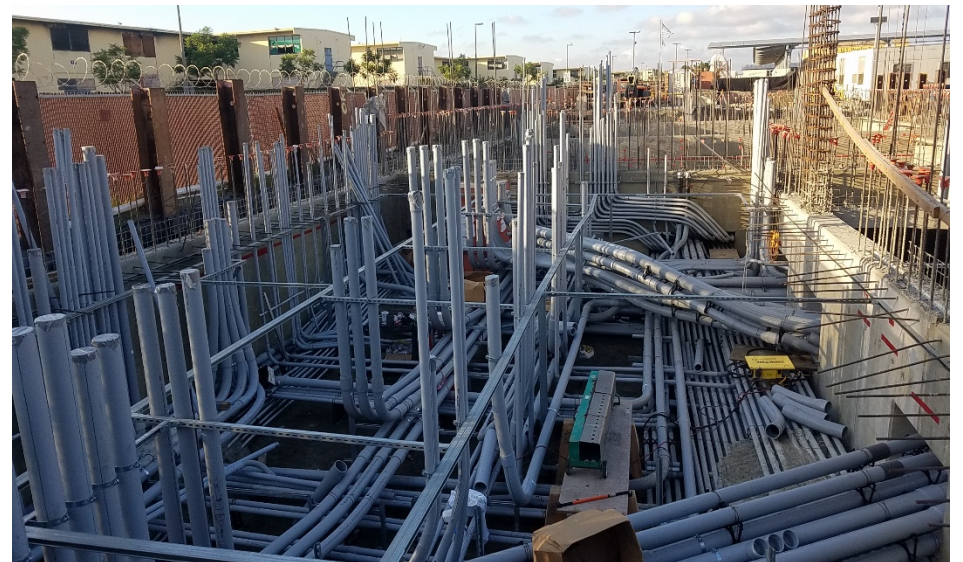
Underslab Conduit in Electrical Room-8 – 10/05/2018
