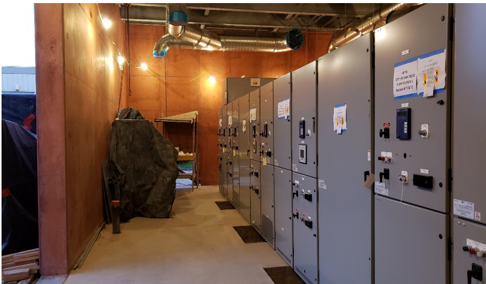
Installation of Switchgear 3 – 09/04/2019
