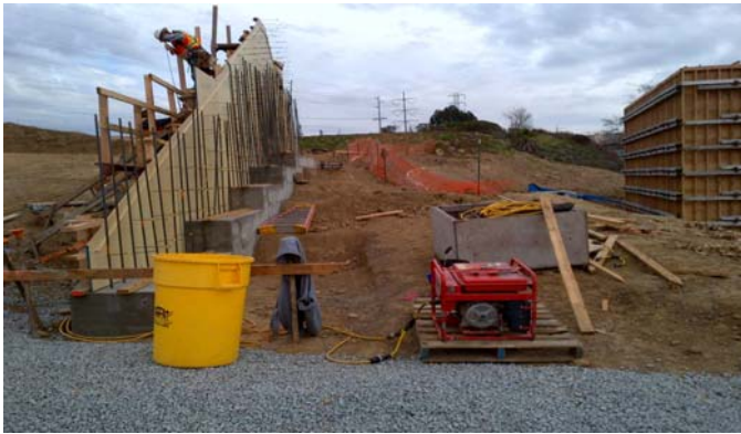
Construction of retaining walls to protect existing SDG&E vaults (R) and to support the new access road to the cogeneration facility expansion (L)
