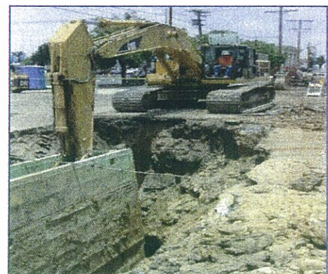
Installation of new 15-inch polyvinyl chloride sewer main along 33 rd Street in Normal Heights.
