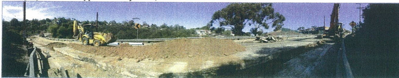
Replacing the 12-inch water main.
