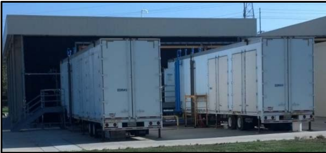
Electrodialysis Reversal trailers at North City Plant
