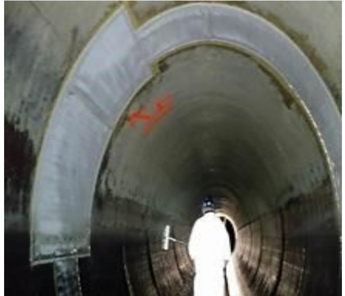
Figure 1 – Before 114-inch West Point Loma Interceptor Pipeline – Before and After Lining repair
