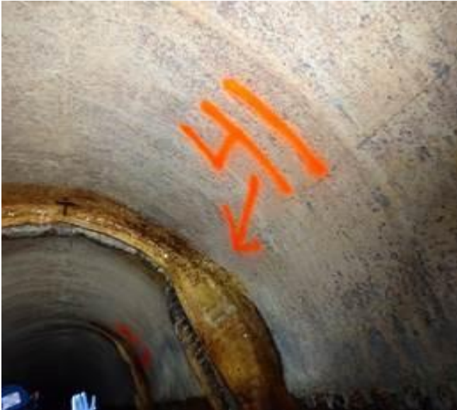
Figure 1 – Before 114-inch West Point Loma Interceptor Pipeline – Before and After Lining repair
