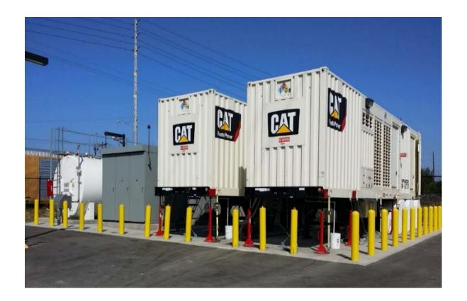
This project purchased seven generators and utilized a design-build contract to install the generators and associated equipment for permanent power connection to existing sewer Pump Stations 1, 64, 65, Penasquitos, North City Reclamation Plant, and Environmental Monitoring Technical Services (EMTS) laboratory.
