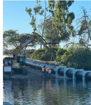
*Construction crews fuse pieces of pipe together on land and string it out on Miramar Reservoir before installing it on the lakebed.*
