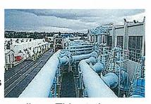
flow into Pump Station #2 is approximately 180 million gallons. This station pumps the wastewater to the Point Loma Wastewater Treatment Plant through two 87" force mains. The two pump stations have 24-hour staffing.
