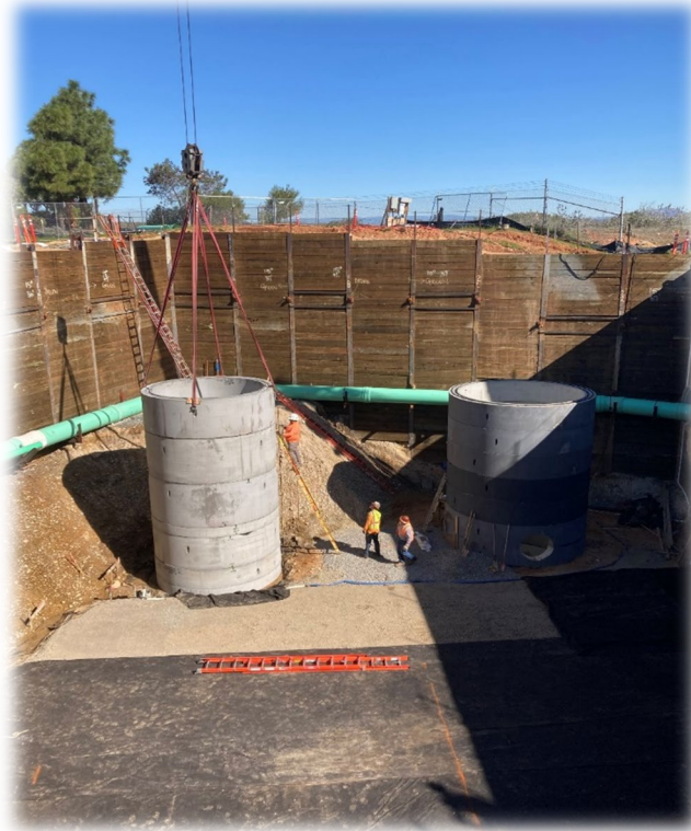
Figure 1. On the left, installation of the Hydrodynamic Separator (10' diameter), the Hydrodynamic separator will remove sediment out of incoming storm water. On the right, the contractor has installed the first bottom rings of the wet well structure (17' diameter).
