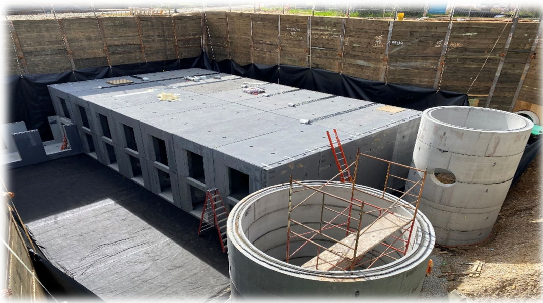
Figure 2. Placement of the second row of the underground storm water storage structure (48'x56'x15').
