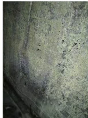
View of seam and bubbles on vertical wall in main structure.
