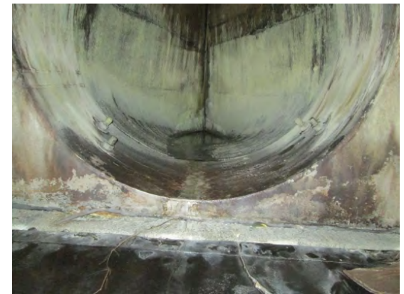
View of interior of 'duckbill' valve and overflow box structure.
