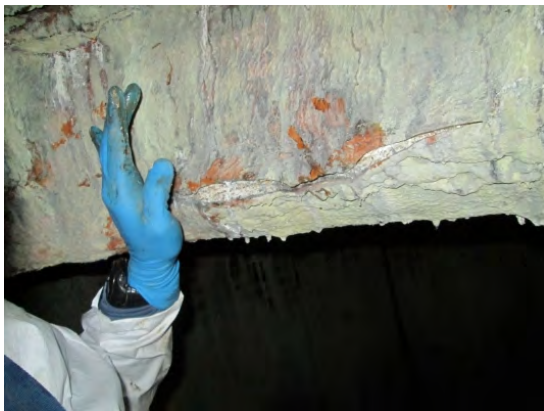
View of cuts in liner at bottom of short barrel section in manhole.
