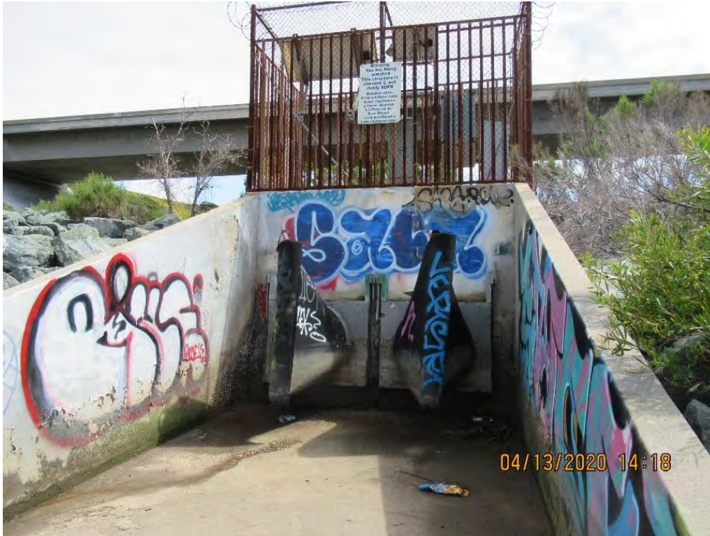
Photo 1. SMI Siphon Transition Structure on the South Bank of the Sweetwater River
