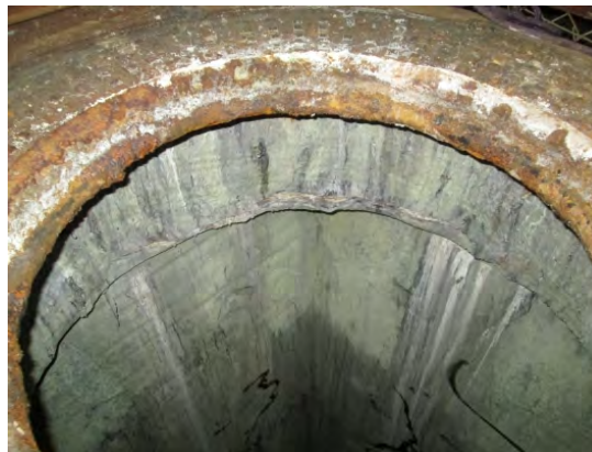
View of corroded manhole frame and cuts in liner at bottom of short barrel section in manhole.
