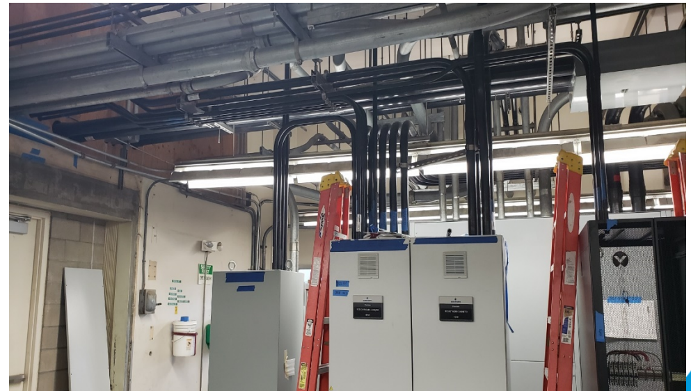
Installation of Control and Signal Conduit Rough-Ins – 06/18/2020
