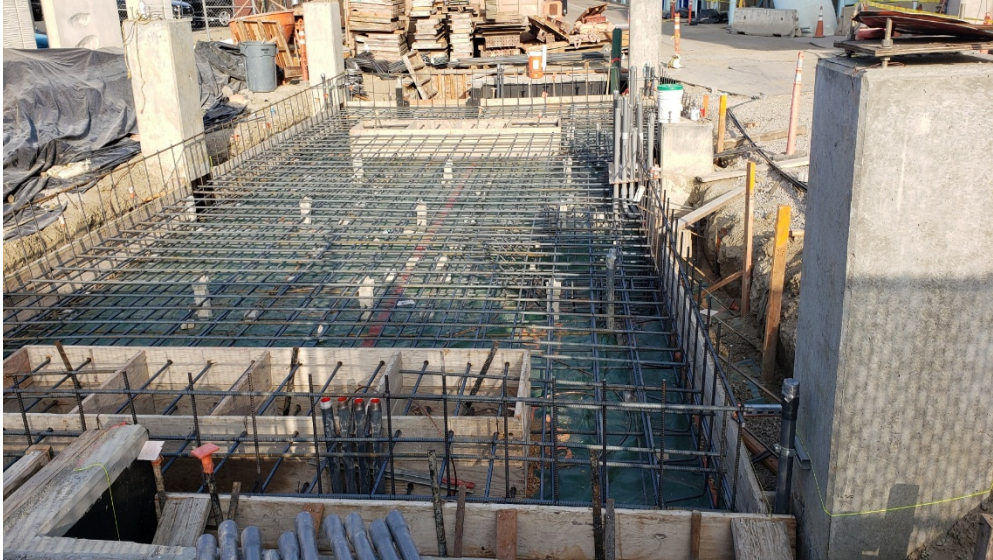
Rebar Work at Fuel Tank Containment Area – 09/26/2019
