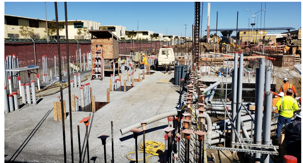
Underslab Conduit in Electrical Room – 02/07/2019
