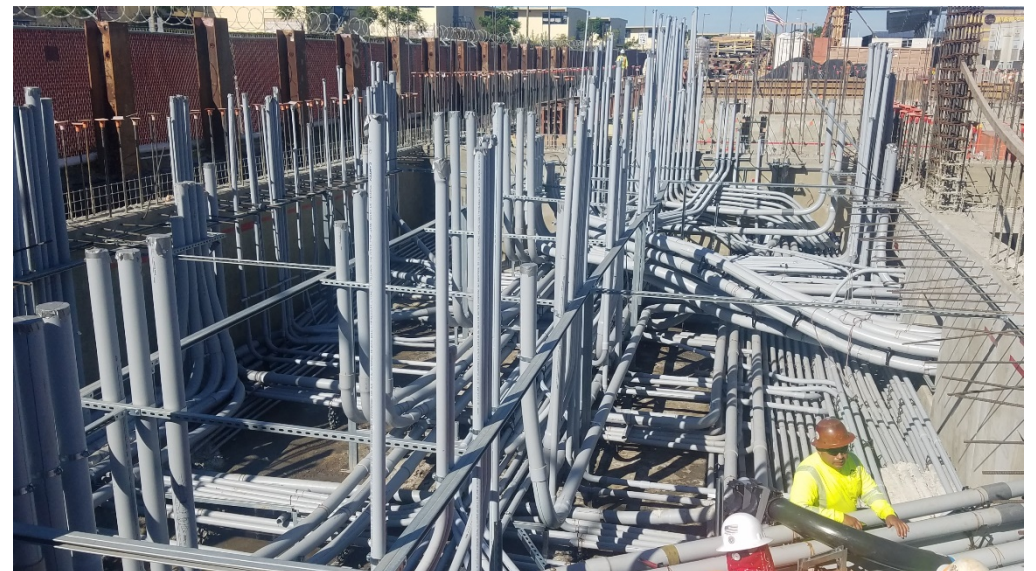
Underslab Conduit in Electrical Room – 10/31/2018
