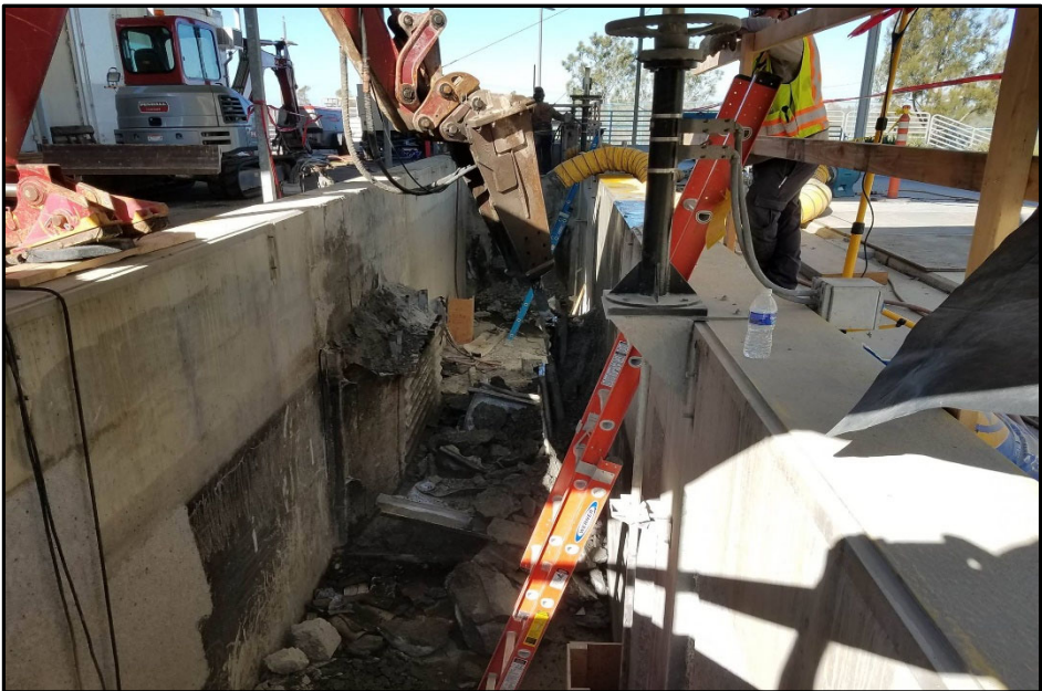
Left Photo: Demolition of the existing UV channel
