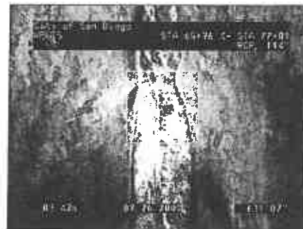
Lining defect from 9 to 3 o'clock, concrete and rebar exposed
