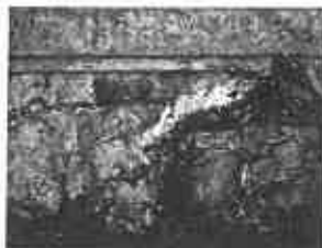
Primary Manhole Grade Ring is Delaminating
