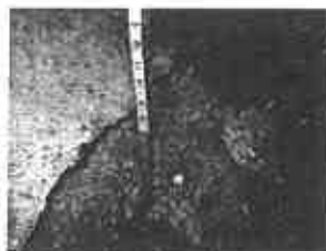
Coating Overhang Caused by Concrete Corrosion
